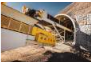
TUNNEL RECLAIM CONVEYOR
